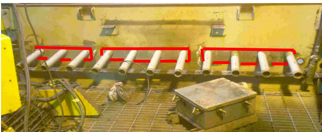
Figure 3. New pipe nipple sections welded into place.
